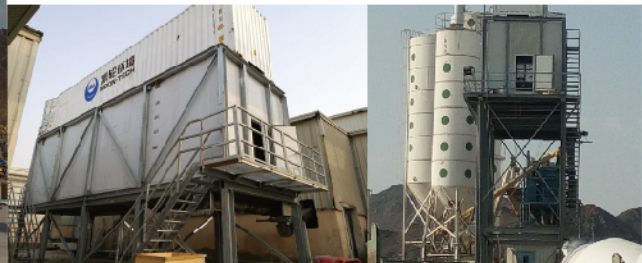
混凝土冷却自动送冰系统 2017 Automatic ice delivery system for concrete cooling 2017
